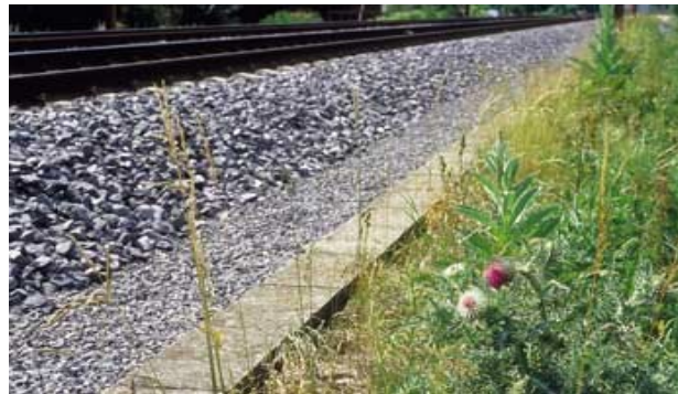
photo 2: concrete bars, Swiss Rail (SBB) 2001
