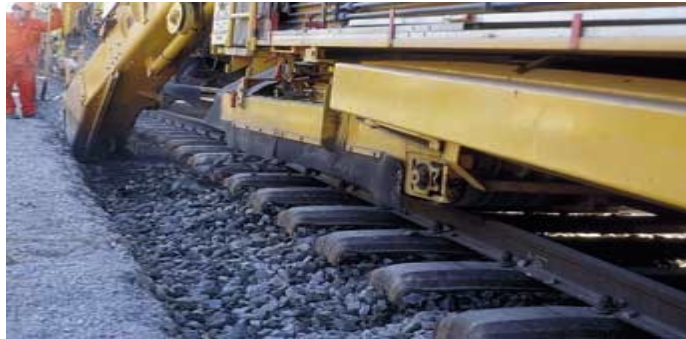
photo 4: ballast cleaning machine (SBB 2001 @ 16)
